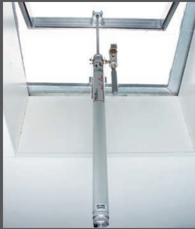
On dome with thermal valve
